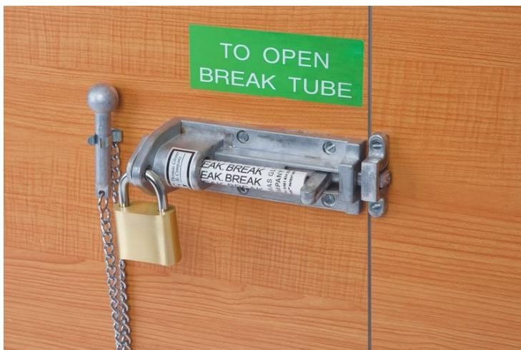
A key in a box, with a breakable cover is not an acceptable locking mechanism for a fire exit door.
